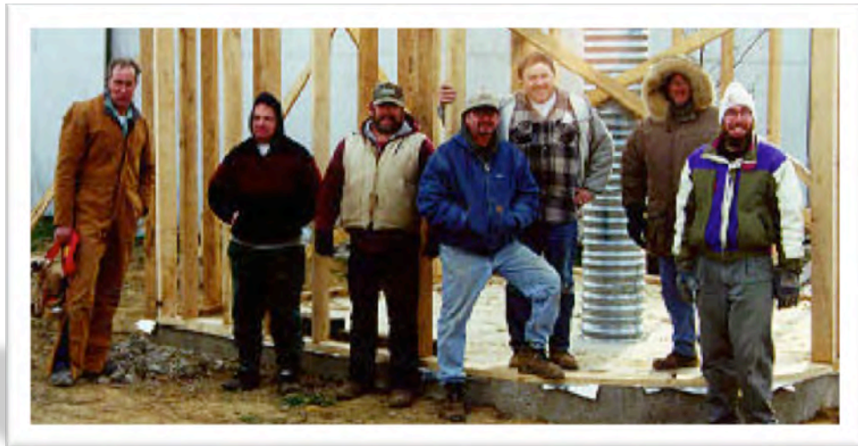
Figure 45. Construction crew working on the Sugar Grove Observatory
